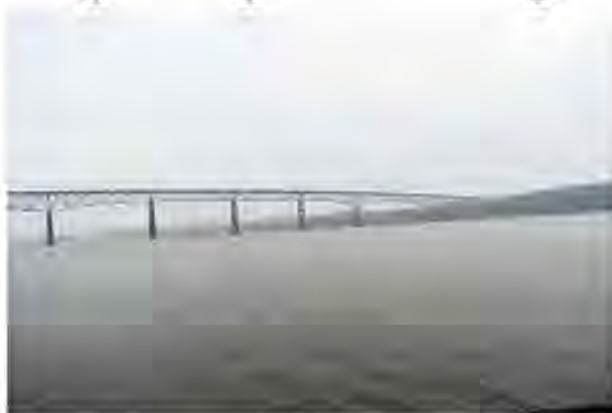
(a) Overview of the bridge's east end from the south
