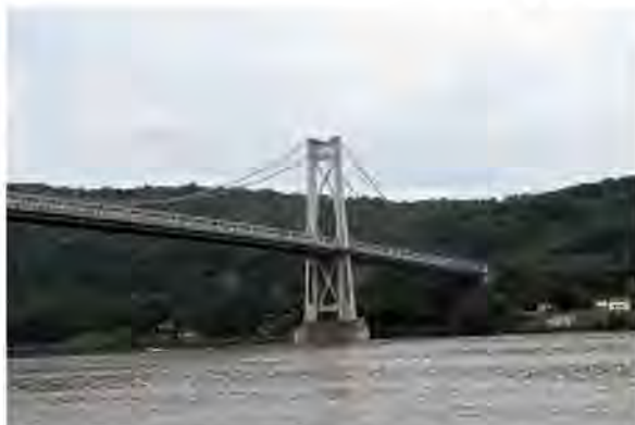
(a) View of the bridge
