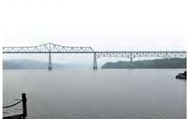
(b) Overview of the mid-span of the bridge
